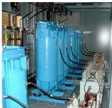
Figure 24: Example for three-phase product with connection in front of coil after assembly
